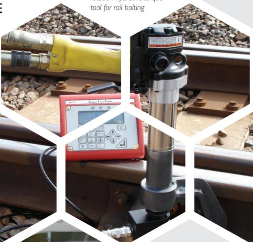
Prototype continuous rotation hydraulic torque tool for rail bolting
