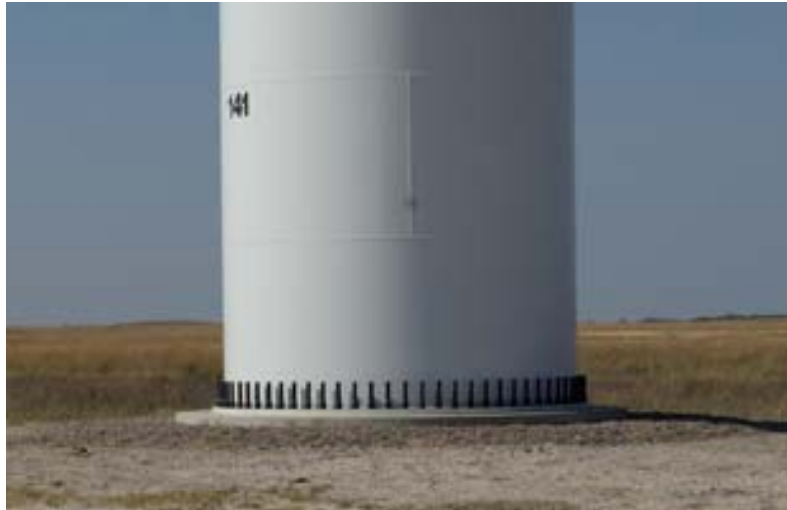
Foundation bolts on wind tower
